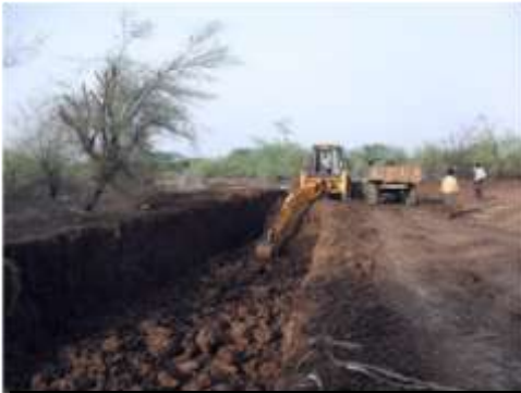
Digging machinery excavating silt from the tanks
